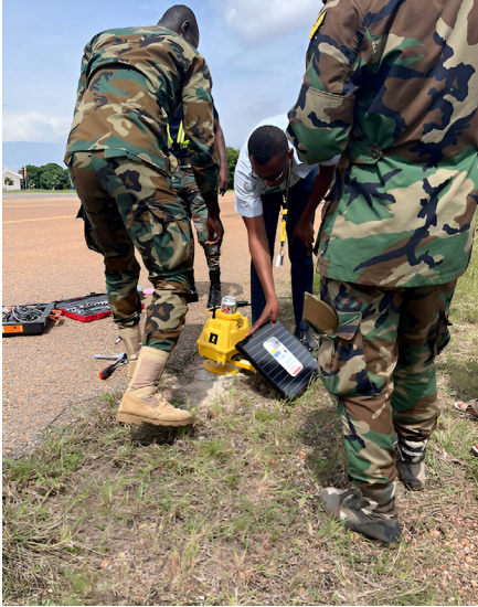
Deployment of S4GA solar airfield lighting, Africa
